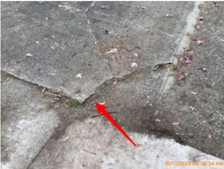
At end of driveway
