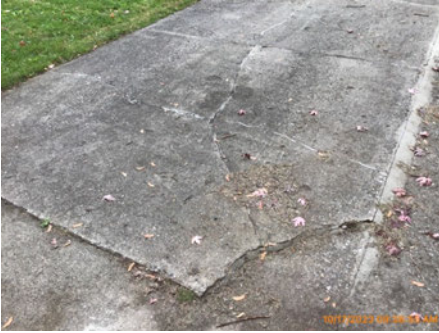
Cracks have been filled
