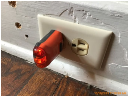
Rear room off of bathroom eastern wall
